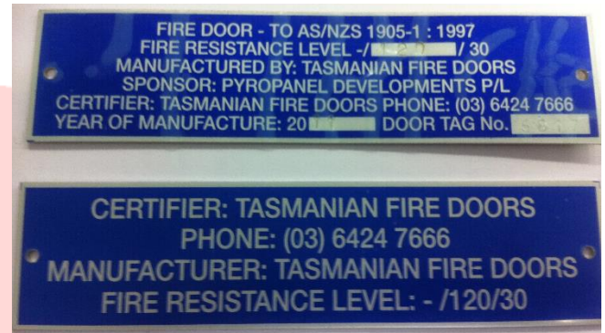
Example of a fire door tag showing fire resistance level
